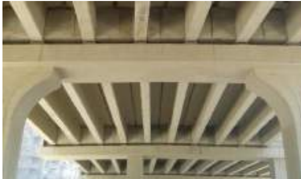
Figure 1: Wide shallow beams application in bridges
