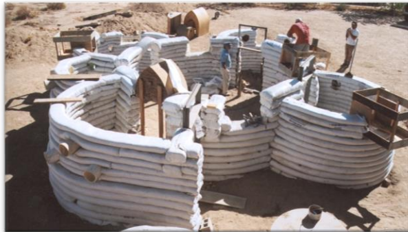
Figure 6-Construction with sandbags, Reference: Sandbag Shelters World Habitat
