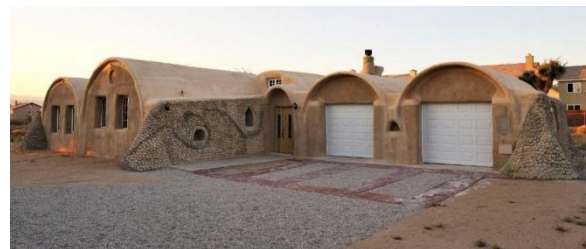
Figure 14-elevation- Resistant Super adobe Reference Super Adobe Structures at Cal-Earth ideas earth bag homes, earth homes, earth ship
