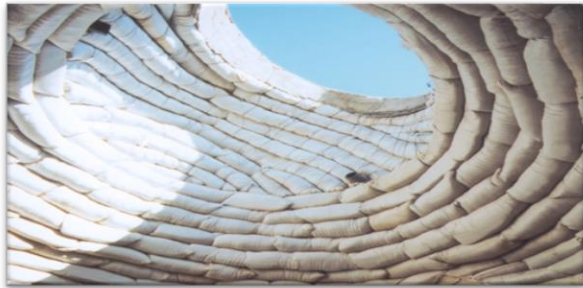
Figure 5-Construction with sandbags, Reference: Sandbag Shelters World Habitat
