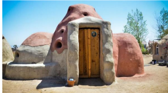
Figure 10-Resistant Super adobe Reference Cal-Earth Makes Disaster-Resistant Super adobe Construction a Reality
