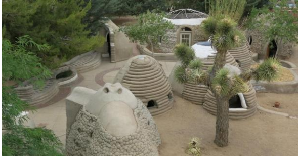
Figure 12-layout- Resistant Super adobe Reference : Cal-Earth Makes Disaster-Resistant Super adobe Construction a Reality
