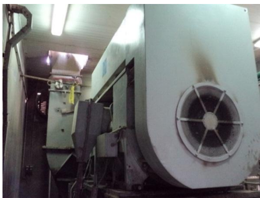
Fig. 2 Photographic image for atomization air blower
