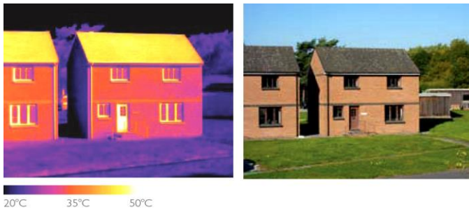
Fig. 30 Images of the houses built to the Swedish building fabric standards. After completion, high temperatures were observed during the day as a result of simulated internal gains and solar gains [7].
