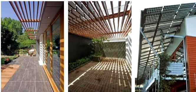
Fig. 28 There are a variety of approaches that may be taken when providing solar shading to a home. These include creating an overhang by the building form along with retractable awnings and external louvres [18].
