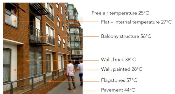
Fig. 32 Thermographic images show the high temperatures of the external surfaces of the apartment building and its immediate surroundings because of their direct exposure to the sun. Air introduced into the flat by opening windows will therefore be significantly warm [25].
