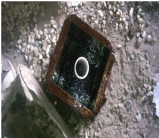
Fig (3) Preparation of hollow core in concrete cubes
