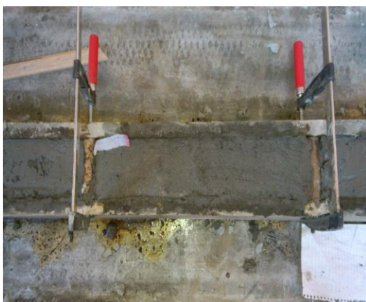
Fig (5) Concrete beams during casting
