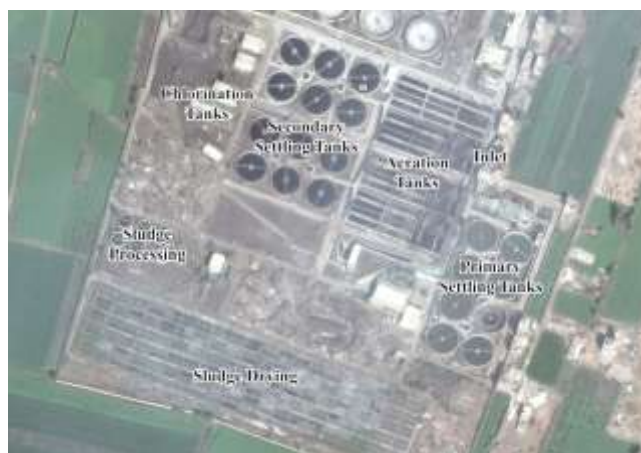
Fig. 5. Mansoura WWTP description
