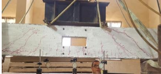
Fig. 7c Crack pattern for CBMO
