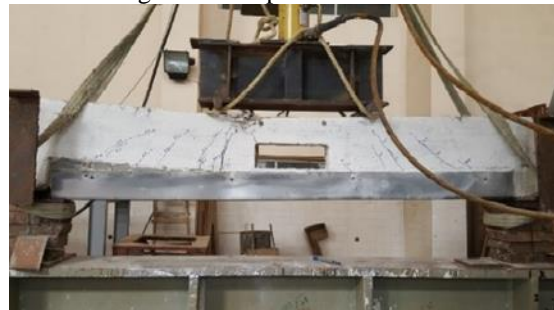
Fig. 9b Crack pattern for BMOST2
